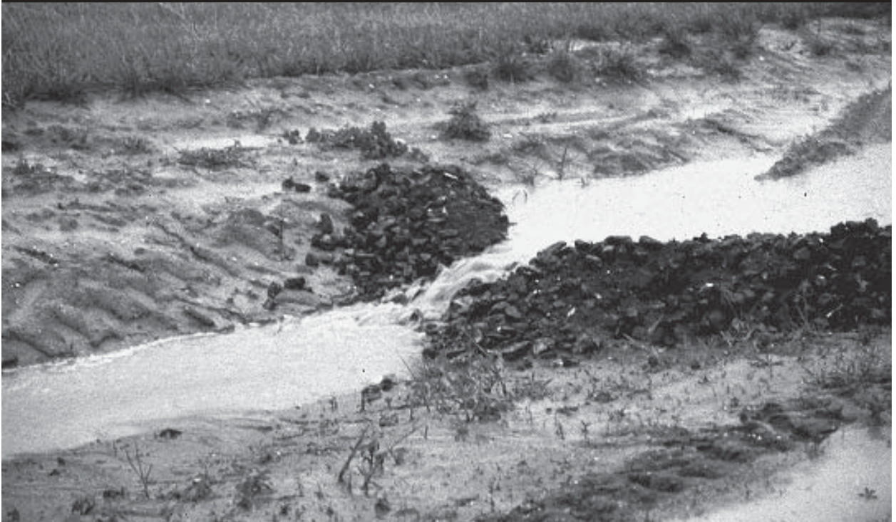
Plate 1.4 Rock Check Dam
